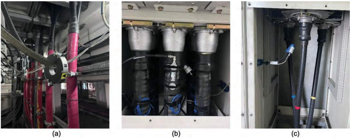
Figure 2. Installation of sensors and positioning for (a) a high-frequency-current-transformer sensor on the ground lead, (b) TEV sensor on the cable, and (c) ultrasonic airborne sensor.
